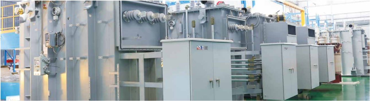
9 Units 20MVA 13.8kV Delta to 25kV GrdY Substation Transformers for Oil&Gas Projects for TX, USA
